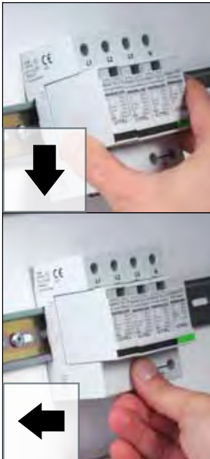
Slide the top of the surge protector onto the rail, and press the bottom until the unit snaps into place.
