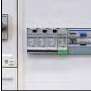
Example of a DS Series application in a standard electrical cabinet in compliance with international standard.
